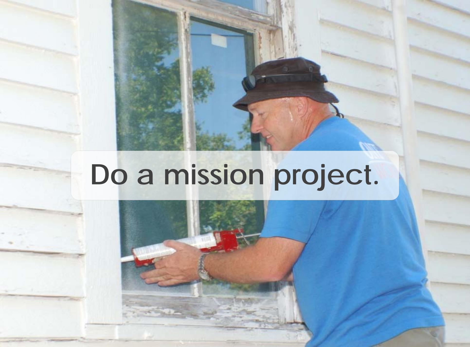
A man wearing a blue t-shirt, a brown bucket hat with sunglasses on top, and a watch is using a red caulk gun to seal the bottom of a window frame. The house has white horizontal siding. The window is partially open, and the man is looking down at his work. A semi-transparent white box with black text is overlaid on the image.
